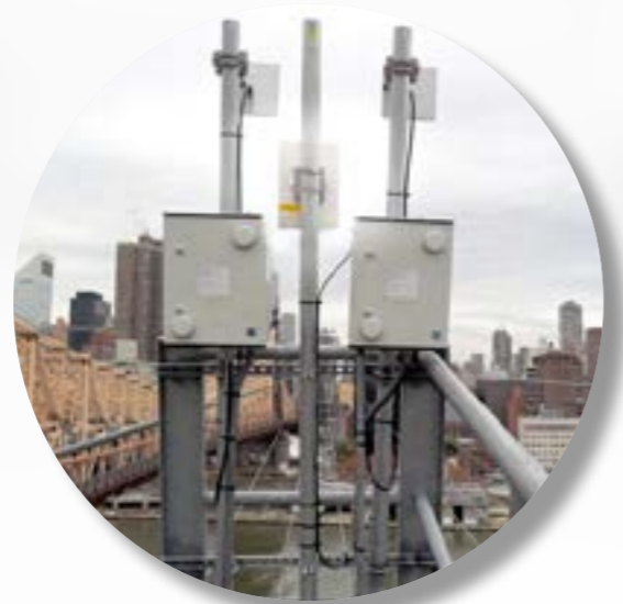
2. DATAEAGLE Classic 3702A in the protection cabinet at one of the two cabins.
