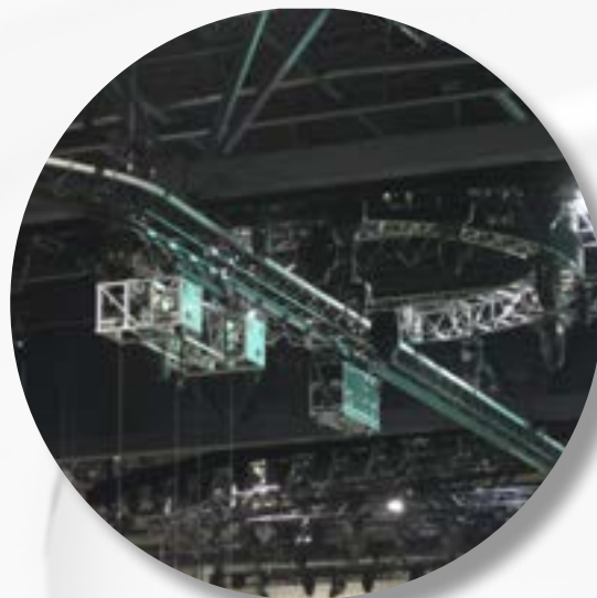
2. Via this rain construction the bird is controlled accompanied by the power electronics with DATAEAGLE .
